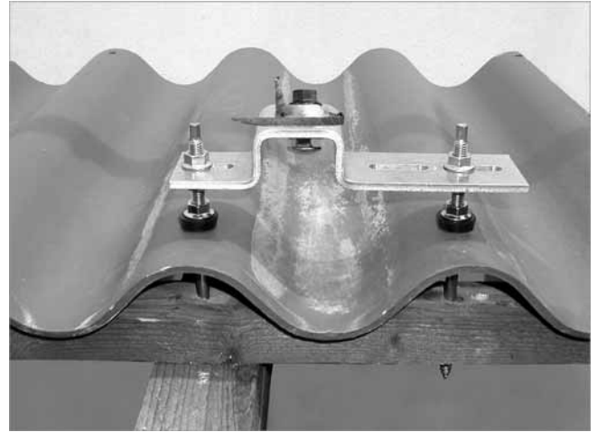
Fig. 19: Installed roof-mount frame (Method B)
